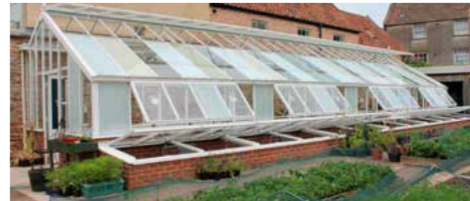
Greenhouse at The Bishop's Palace, Wells, painted with opaque colours for intense shading on roof panels and decorative stencil designs + White Witch on wall windows
